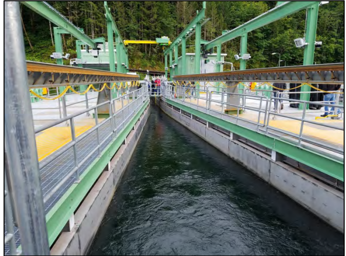
PGE’s River Mill Dam floating surface water collector for juvenile salmon, steelhead, and Pacific lamprey out-migrants. Source: John Runyon, Cascade Environmental Group
