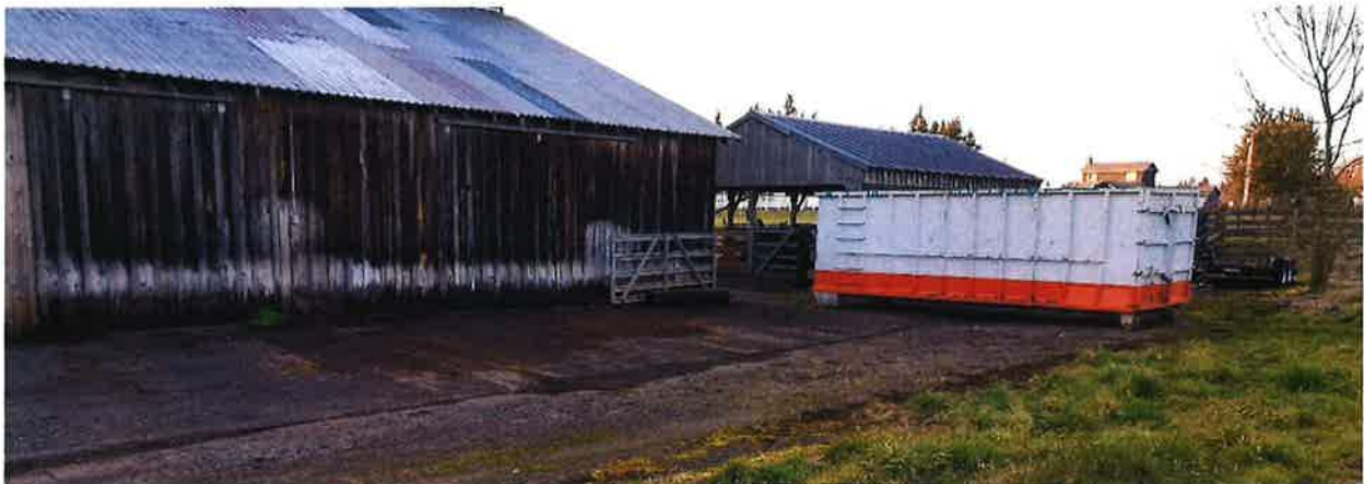
The same area following debris removal
