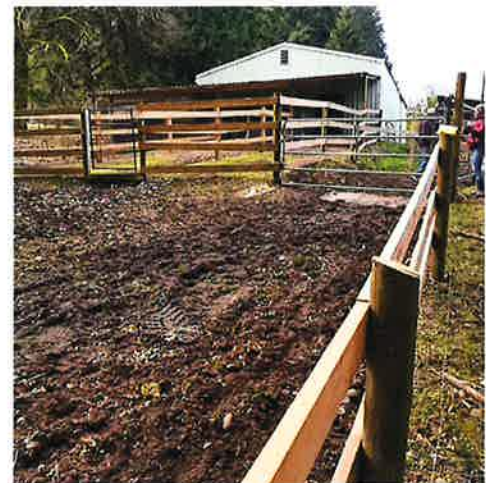
Muddy paddock before construction.
