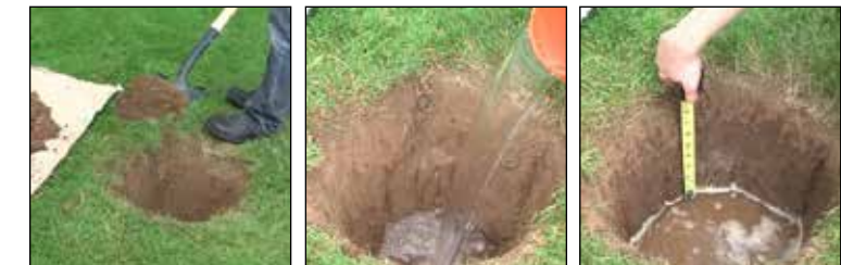
Dig a test hole 24" deep and 12" wide
