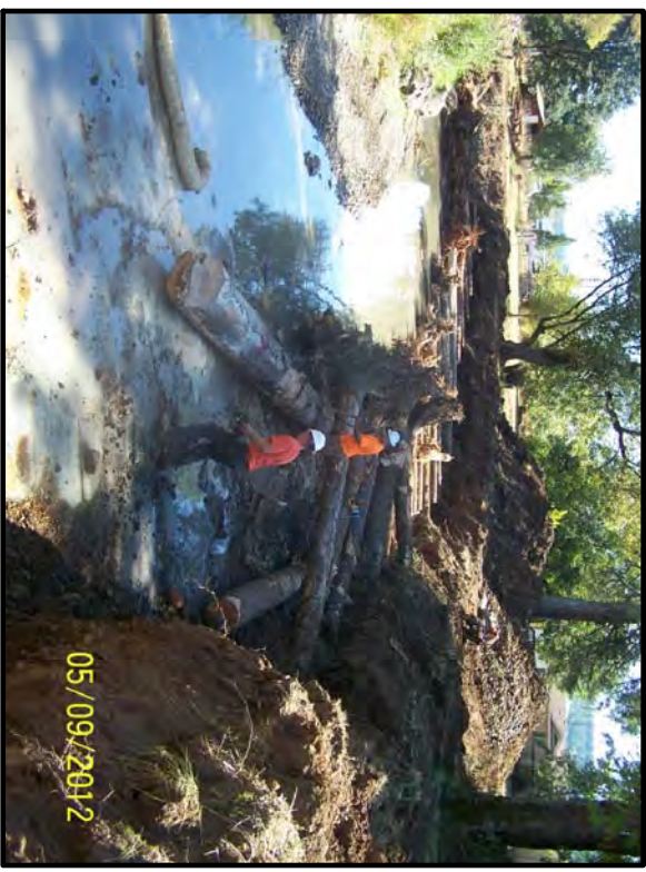
Looking upstream at base members and deflector rootwads
