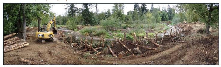
Our big story for this edition of Conservation Actions is the installation of a streambank protection and habitat improvement structure that is 388 feet long! This is one of the largest projects we've undertaken. By persevering and remaining flexible, we overcame obstacles and finished installing the structure in September.
