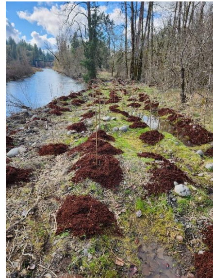
Left: Looking up-river at Barton Natural Area in Spring of 2024 after Fall in-stream construction. Right: 16,000 native trees and shrubs planted post in-stream construction at Barton Natural Area. Mulch rings were installed to help plants survive in the rocky conditions found on site.
