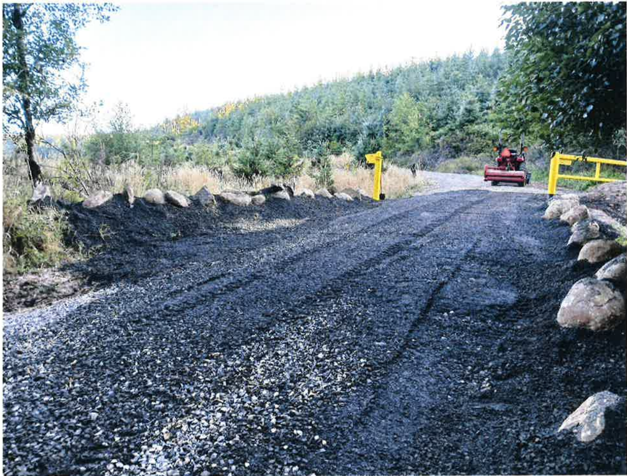
Figure 2 - Boulder placement along entry embankment at the ECCF
