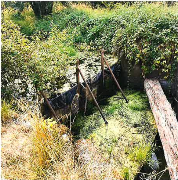
Rock Creek push up dam.
