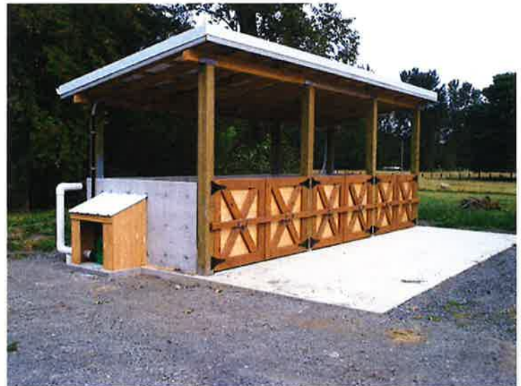
An example of manure composting system the District helped install.
