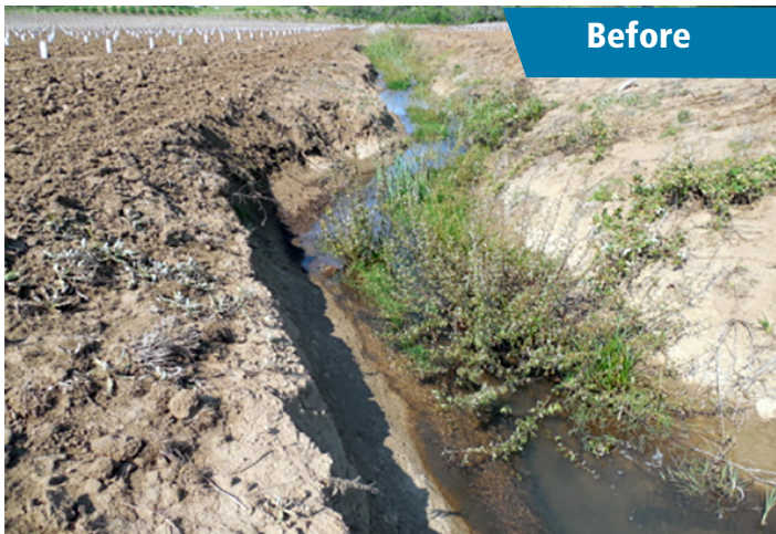
Photo is of a year-round stream in the Willamette Valley. Agricultural activities prevented the ongoing growth and establishment of streamside vegetation, which put this operation out of compliance with Area Rules. ODA photo
