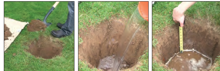
Dig a test hole 24" deep and 12" wide Fill the hole with 8-10" of water Measure drop in waterline per hour
