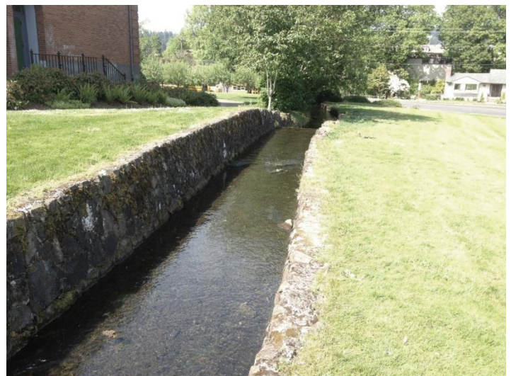
This urbanized stream is not fish friendly!
