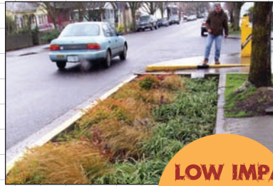
Bioswale with native plants in parking strip absorbs run-off from sidewalk.
